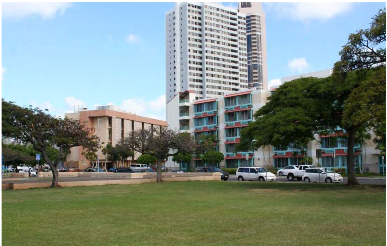
Figure 39. Existing View and Simulation Near Elevated Guideway from within Mother Waldron Neighborhood Park
